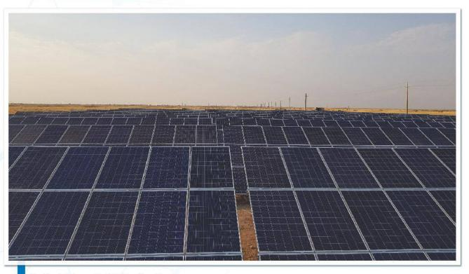
**Buin Zahra 1 MW plant**Double-post design, Three modules in portrait on 4 purlins, Concrete slab foundation
