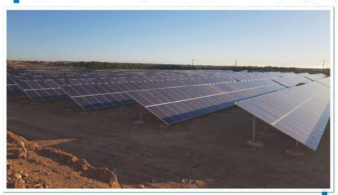
**Shush 1 MW plant**Double-post design, Two modules in portrait, drilling + discrete concrete foundations
