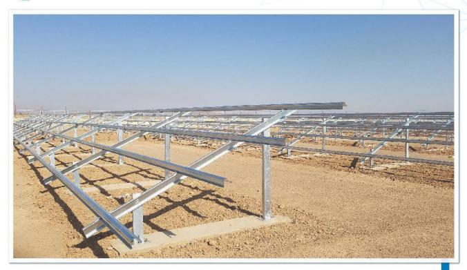
**Talkhouncheh 1 MW plant**Double-post design, Two modules in portrait, Concrete slab foundation
