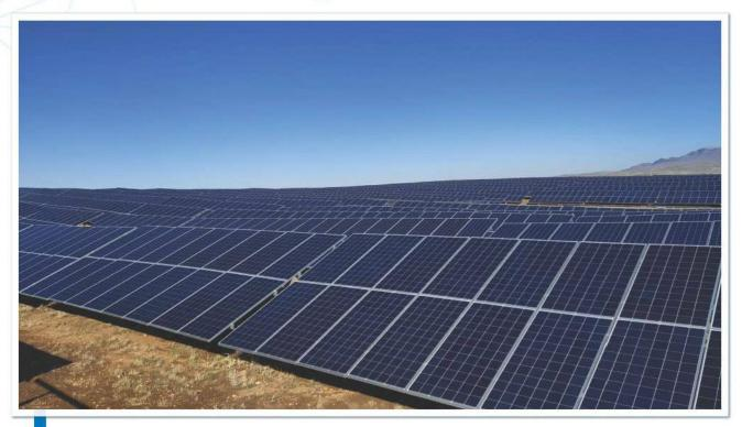
**Kohmarreh 10 MW plant**Double-post design, Two modules in portrait, Rammed piles
