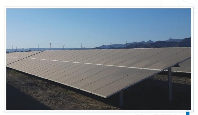
**Kahnouj 5 MW plant**Double-post design, Two modules in portrait, Rammed piles
