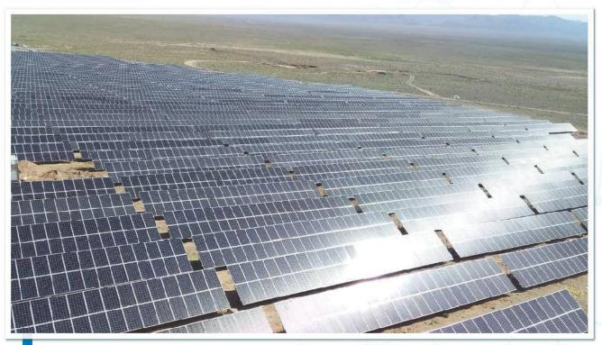
**Sarbisheh 7 MW plant**Single-post design, Two modules in portrait, Concrete pile on uneven terrain
