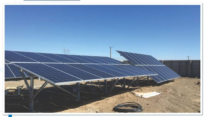
**Marvdasht 1 MW plant**Adjustable tilt single-post design, Two modules in portrait, Concrete foundation
