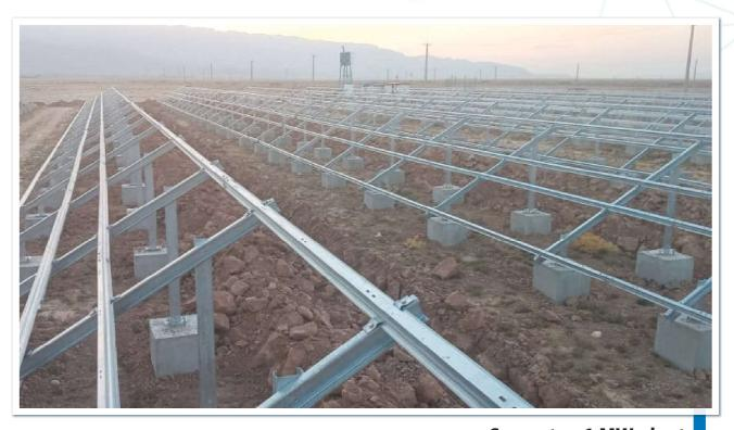
**Sarvestan 1 MW plant** Two-post design, Two modules in portrait, Concrete Slab Foundation
