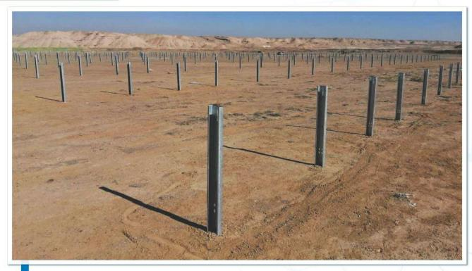
**Hasan abad 5 MW plant (under construction)**Single-post design, Two modules in portrait, Rammed piles
